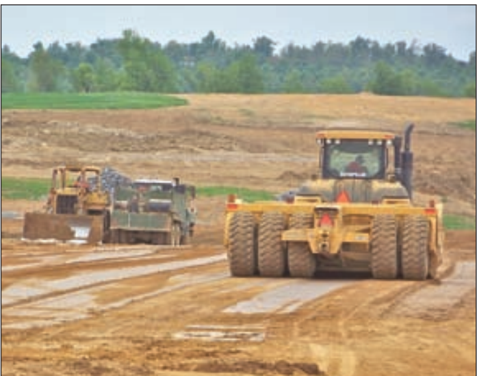
PHOTO BY KEITH TODD, KENTUCKY TRANSPORTATION CABINET Grade and drain work for a four-lane U.S. 641 from Marion to Fredonia continues. A four-lane roadbed will be made, but pavement will only be laid for a super two-lane road.
